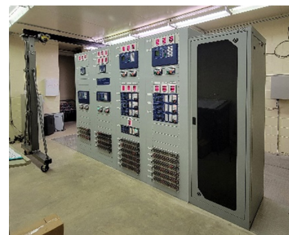
T&D System Upgrades
