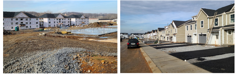
New construction in the borough with natural gas hookup
