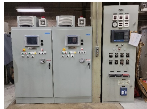
Gen. Controls - Unit 5 (left), Unit 6 (center), Unit 7 (right)
