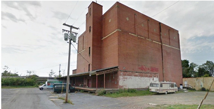
Cold Storage Building on South Fourth Street
