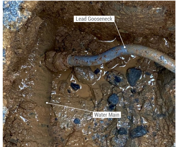
Lead Gooseneck connected at the water main
