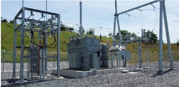
Solar Interconnection Substation
