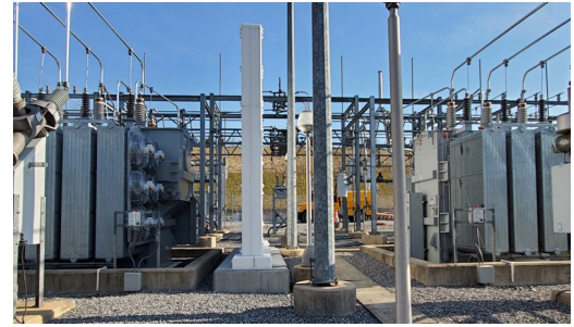
Commerce Street Substation
